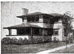
A No. 5-22-W IDEAL Boiler and 447 feet of 38 inch AMERICAN Radiators, costing the owner $235, were used to heat this cottage. At this price the goods can be bought of any reputable, competent Fitter. This did not include cost of labor, pipe, valves, freight, etc., which vary according to climatic and other conditions.
